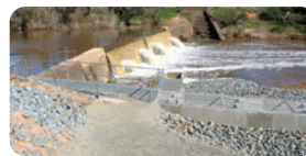
Fishways allow fish to move around barriers such as weirs (JO)
