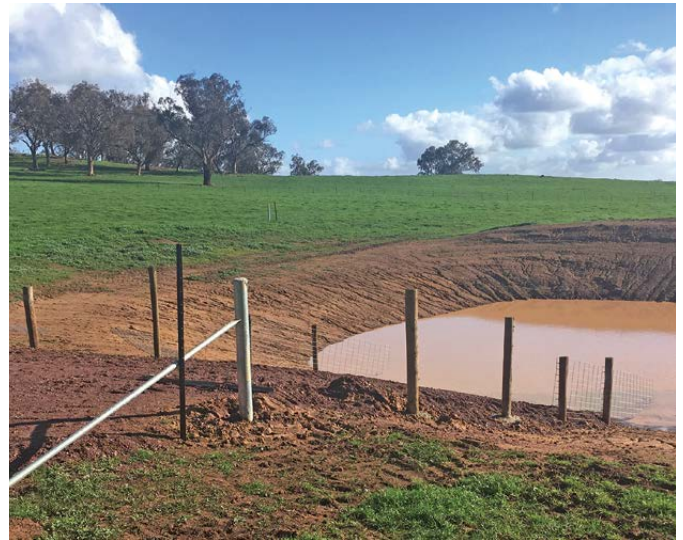
A newly installed hardened access point for livestock. The next step will be to fence around the remainder of the dam perimeter to exclude stock and enable revegetation. (Photo: M. Crane.)
