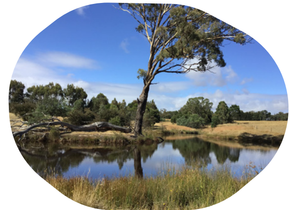
An improved dam on Janet and Justus' property.
